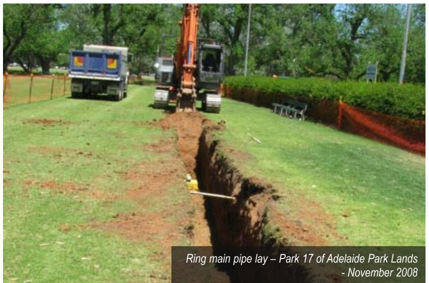
Trunk main pipe lay in Adelaide Airport Land (750mm pipe) – September 2008
